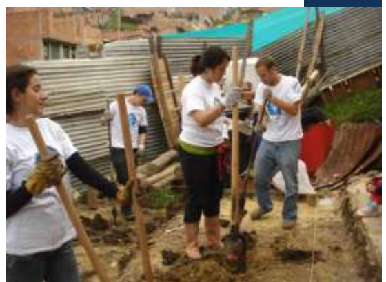
Digging holes for the posts Rincon De Lago, Cauca
